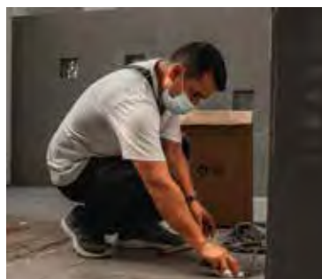
◀ To further prevent mosquito breeding in common areas, anti-mosquito valves are installed in some of the gully traps across the estate.
